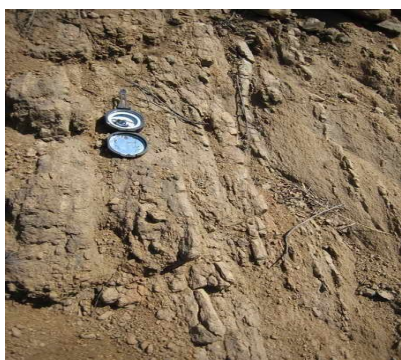
图5 隧道洞口附近构造挤压破碎岩 Fig.5 Tectonic extrusion-broken rocks near entry
