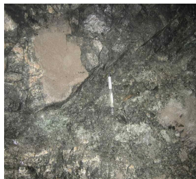
图6 隧道掌子面破碎岩体 Fig.6 Fractured rocks at working face
